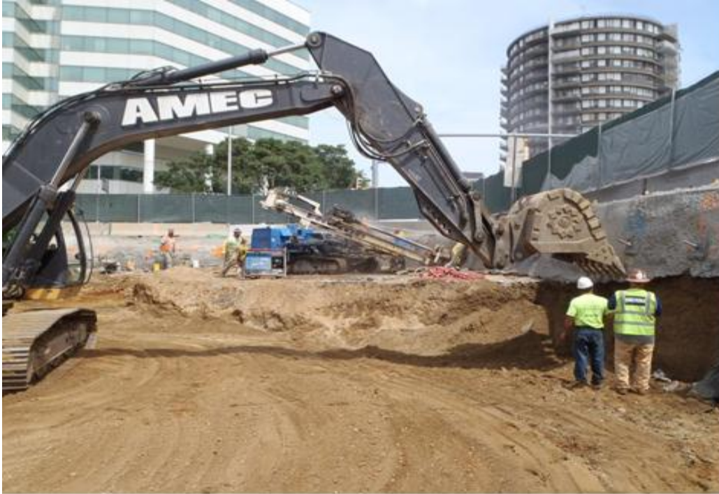
Figure 8: Photo. Excavation of soil lift during construction of soil nail wall.
