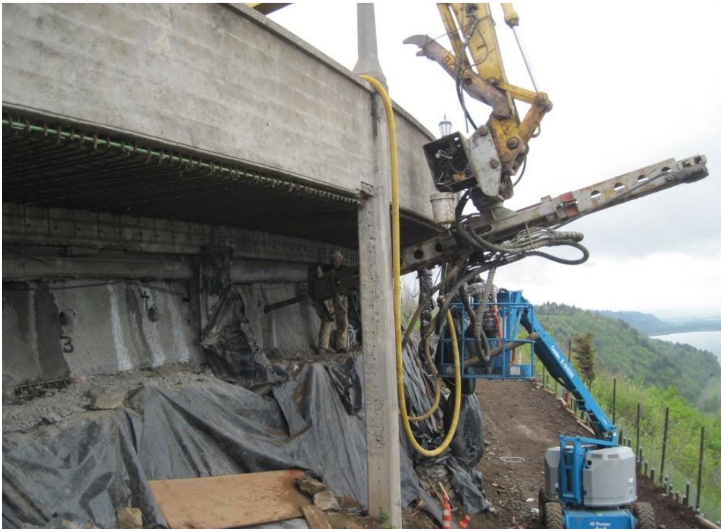
Figure 9: Photo. Drilling Nail Holes.
