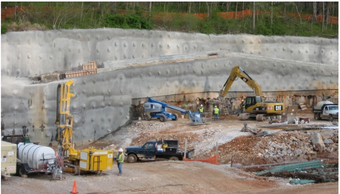
Figure 3: Photo. Construction of Soil Nail Wall
