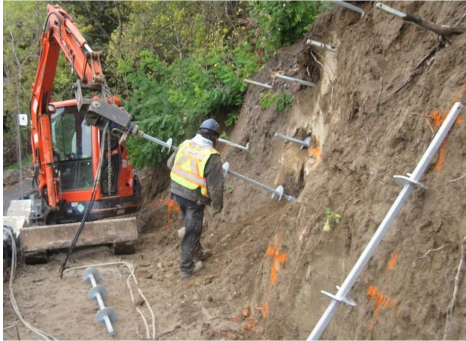
Figure 11: Photo. Screw-in nail installation.
