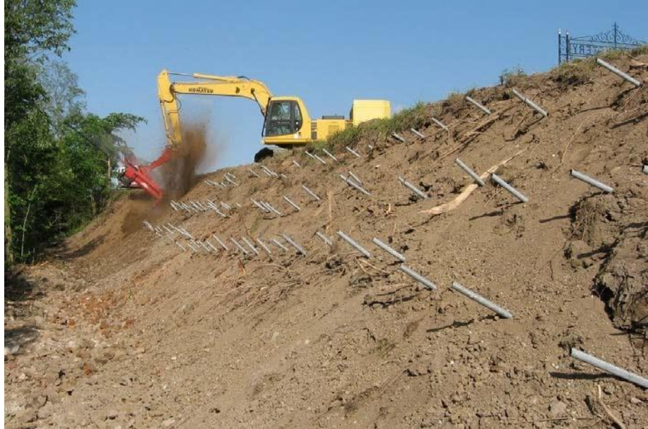
Figure 10: Photo. Launched nail installation.
